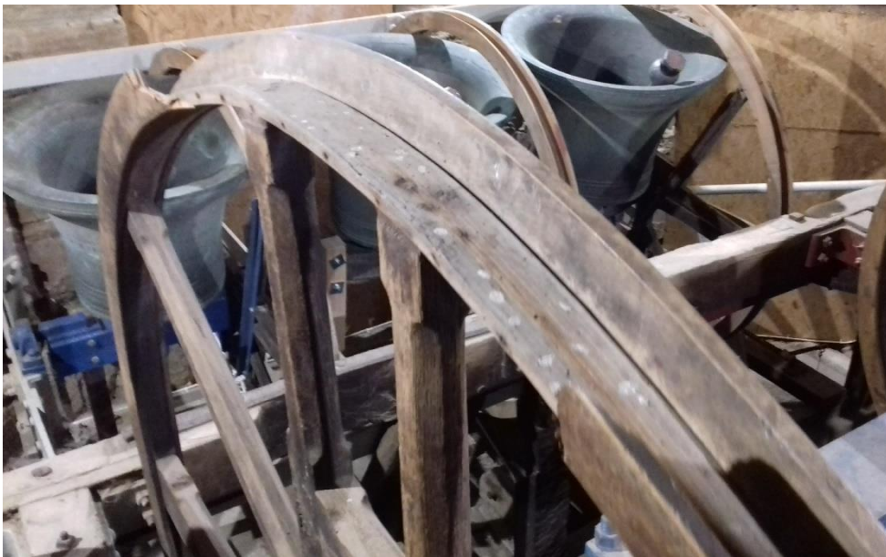
Wear and tear on one of the bell wheels: part has broken away, and there is woodworm here as well as in the main bell frame.
