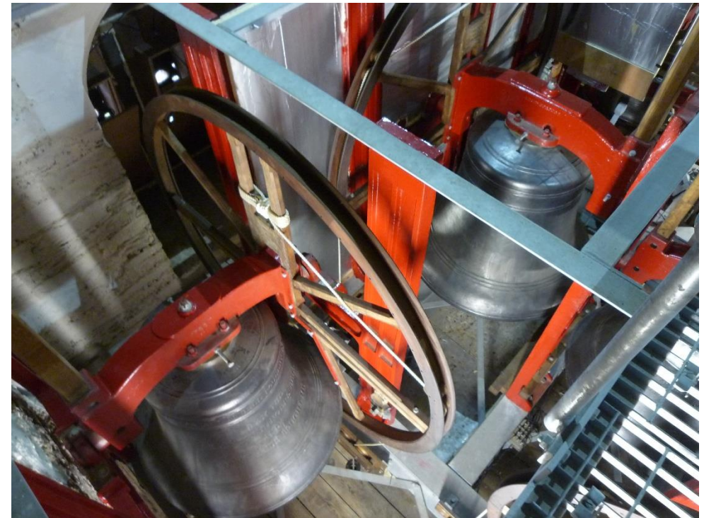
This is what a newly refurbished peal and bell frame can look like, courtesy of St Mary Magdalene church in Taunton, for which 15 new bells were cast in 2016.
